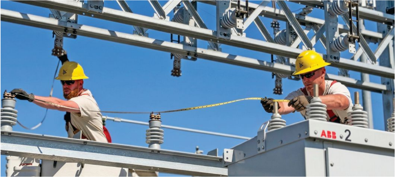
Apprentice Substation Technicians Ryan Howington and Bryan Cutlip work on new equipment at the soon-to-be-energized Millbrook Substation.
